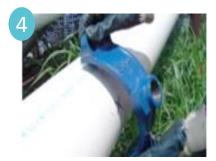
Position the saddle Top on the pipe in the location where it is to be tapped. Rotation of the saddle should be avoided at all times.
