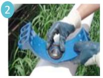
Confirm the PowerSeal Twin Seal saddle gasket is in the proper position in the saddle body.
