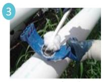
Lubricate pipe and face of gasket with soap and water. For cold weather lubrication, ethylene glycol can be added to the soap solution to prevent freezing.
