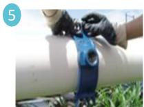
Loosen nuts to the end of the bolt and install saddle Back (s), around the pipe and through the saddle body bolt opening.
